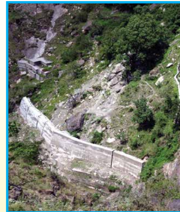
Stabilization of Nigulsari Area
