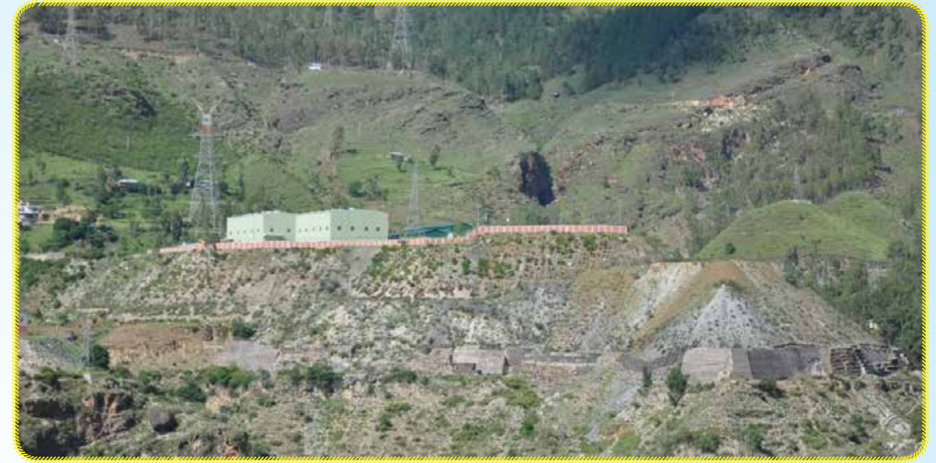
Dumping Site IV on the Right Bank with Restoration Works
