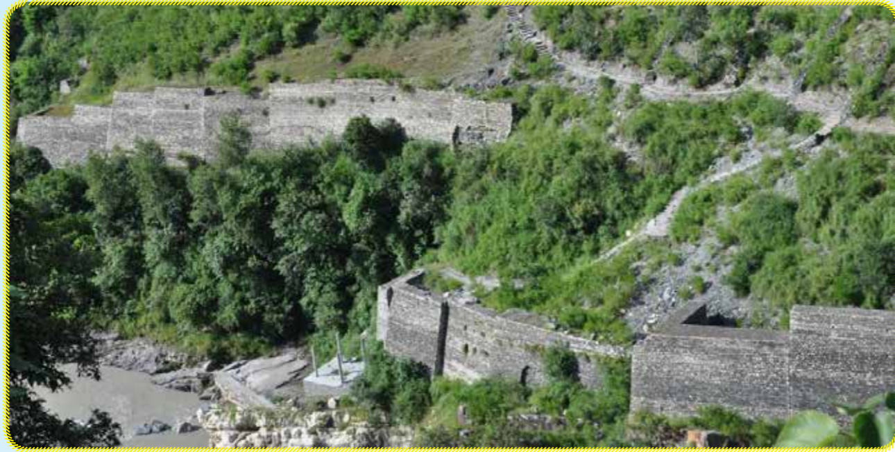
Dumping Site II with Restoration Works
