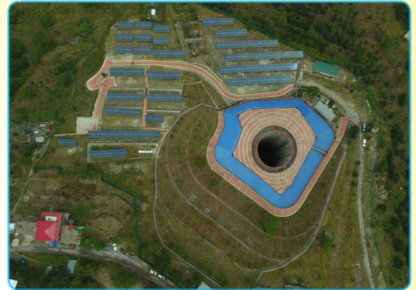
310 KW DC Solar Plant at Surge Shaft
