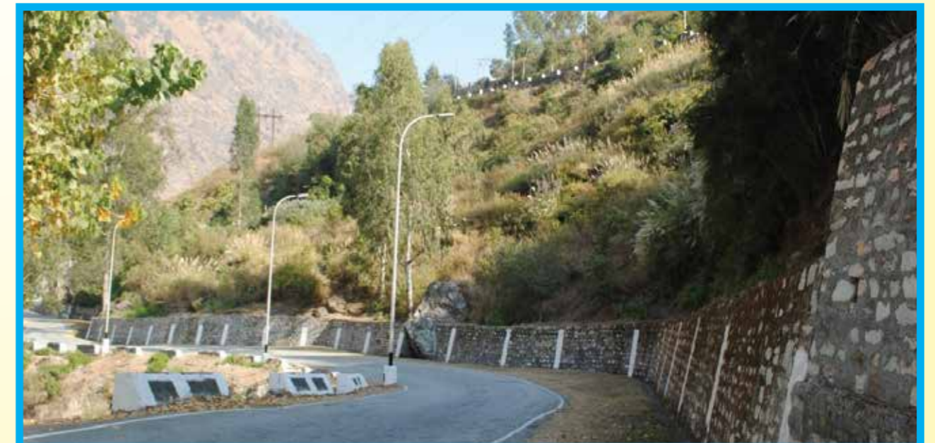
Plantation site along Power House Road
