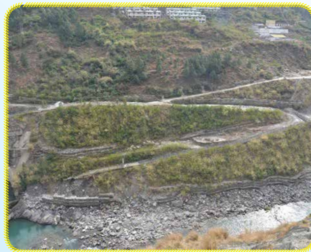
Slope Statbilization Near Spill Tunnel – Jhakri
