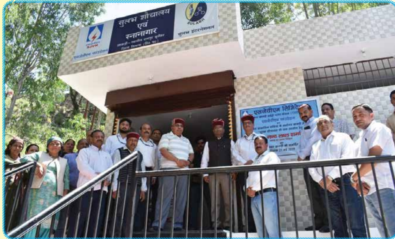
Handing over of Public toilets by Hon'ble CMD, SJVN to Gram Panchayat Jhakri.
