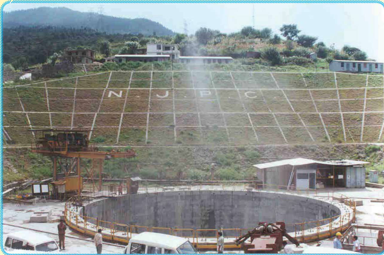
Soil Stabilisation Near Surge Shaft
