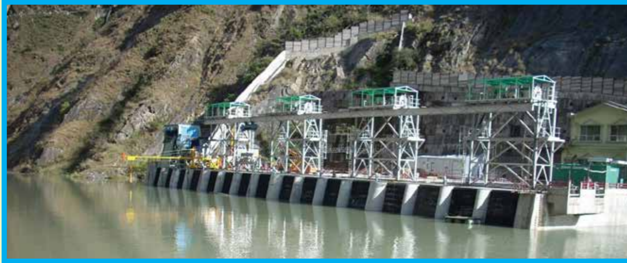
Nathpa Dam Intake Structure
