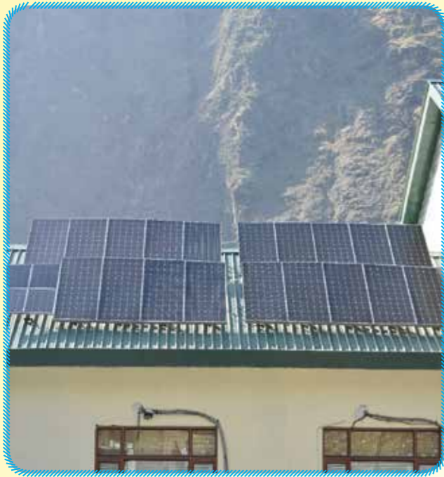
Solar Panels on Office Roof Tops
