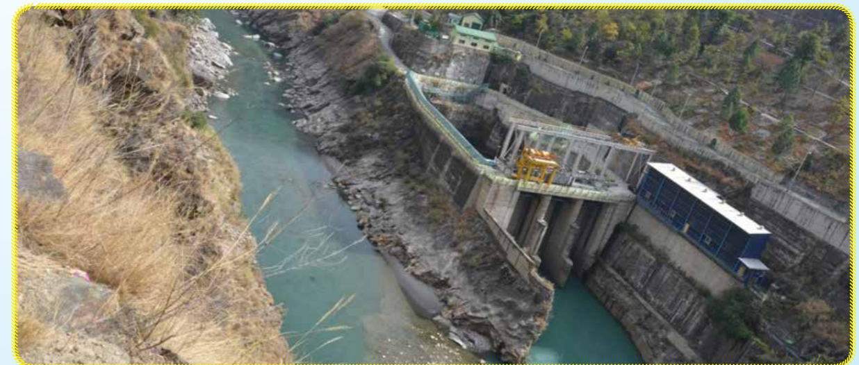
Intake Structure on Left Bank
