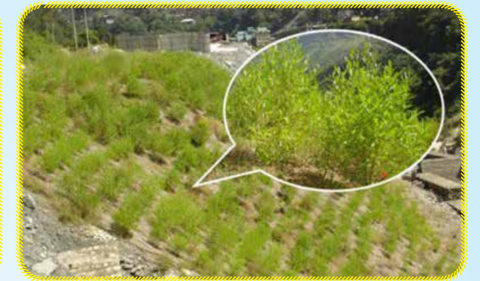
Restored Area After Geo-Green Erosion Control Blanket Technique
