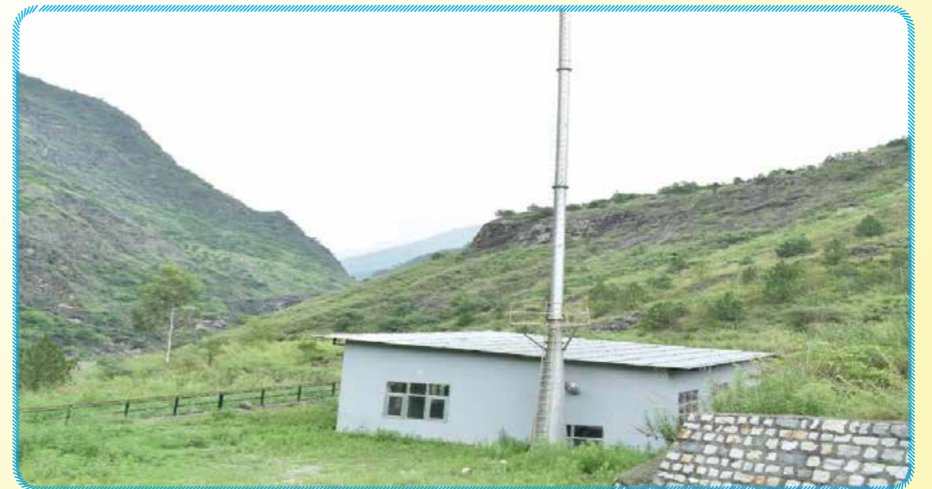
Incinerator Plant at NJHPS
