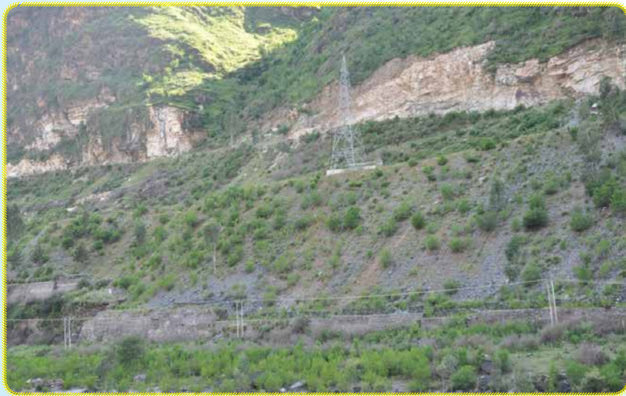
Dumping Site -III on the Right Bank with Restoration Works
