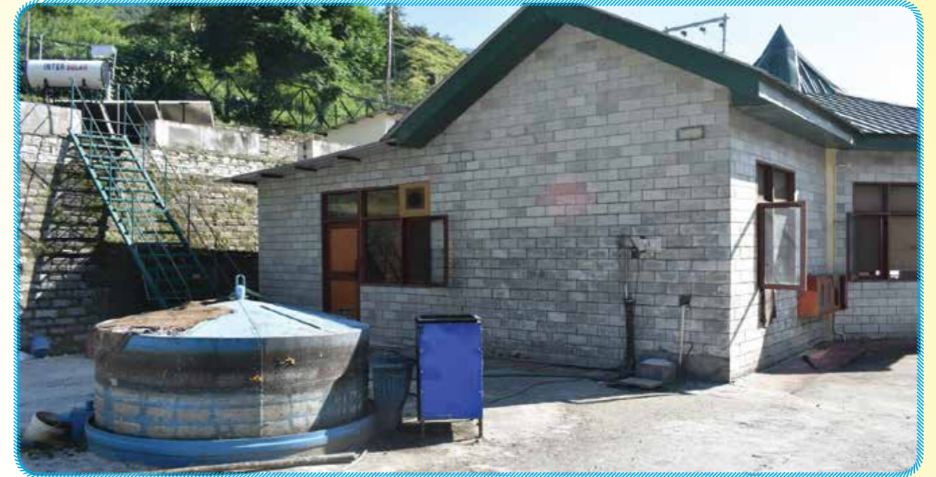
Biogas Plant for Office Canteen, Jhakri
