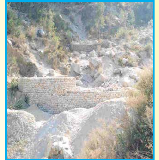
Construction of Check Dam
