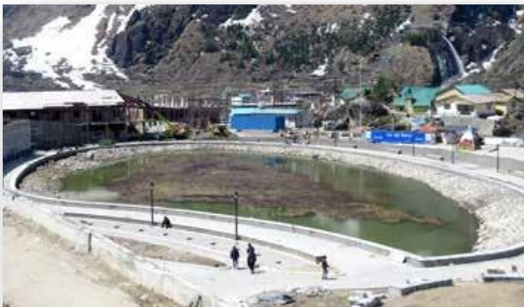
Construction and re-development of Sh. Badrinath Dham (Sheshtra Lake) town as spiritual Smart Hill Town
