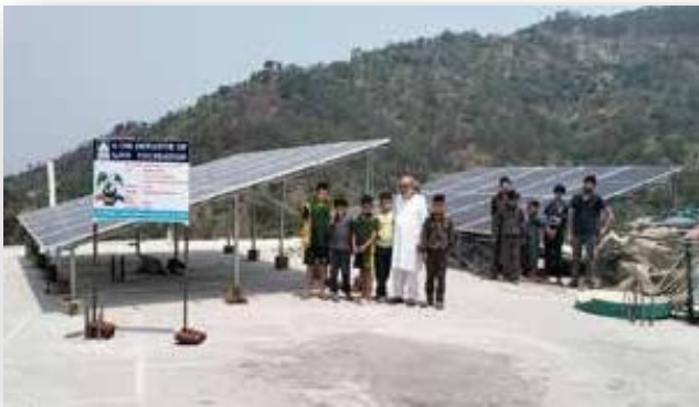
Installation of Roof top Hybrid Solar Power Plant at Deen Bandhu Sewa Mandal Bharnal Distt. Mandi (H.P.)
