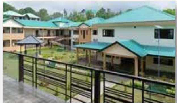
Construction of Senior Citizen Home at Palampur (H.P.)
