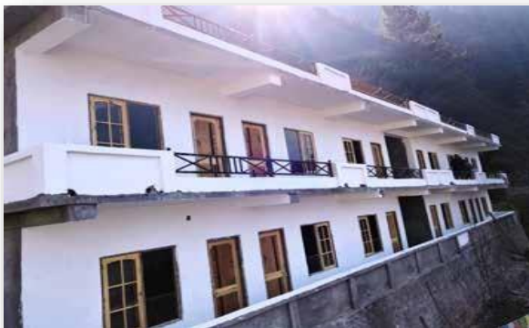
Construction of Hostel-cum-meditation centre at Rin Gchen Zangpo, Endowment Society, Ponda Distt. Kinnaur
