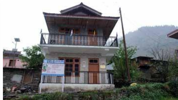
Renovation of Community Hall at Village Majhewali in Gram Panchayat, Funja Tehsil Rampur Distt. Shimla H.P.
