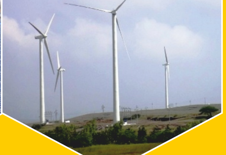
47.6 MW Khirevire Wind Power Project of SJVN
