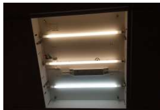
Conventional T-5 FLT Recessed Mounted Light Fixtures with choke installed in SJVN
