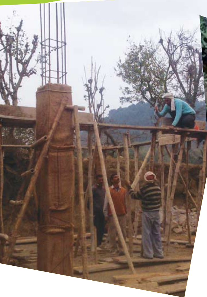
Construction work at GMS Jeehan- DSHEP
