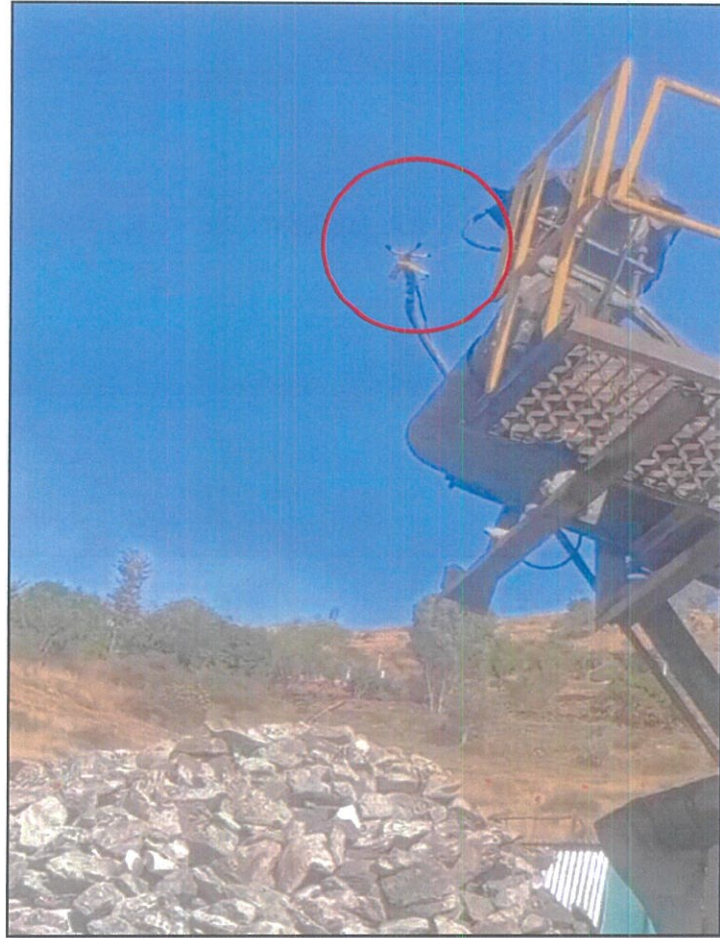
Picture-3. Water sprinkler being used at Crusher Plant.
