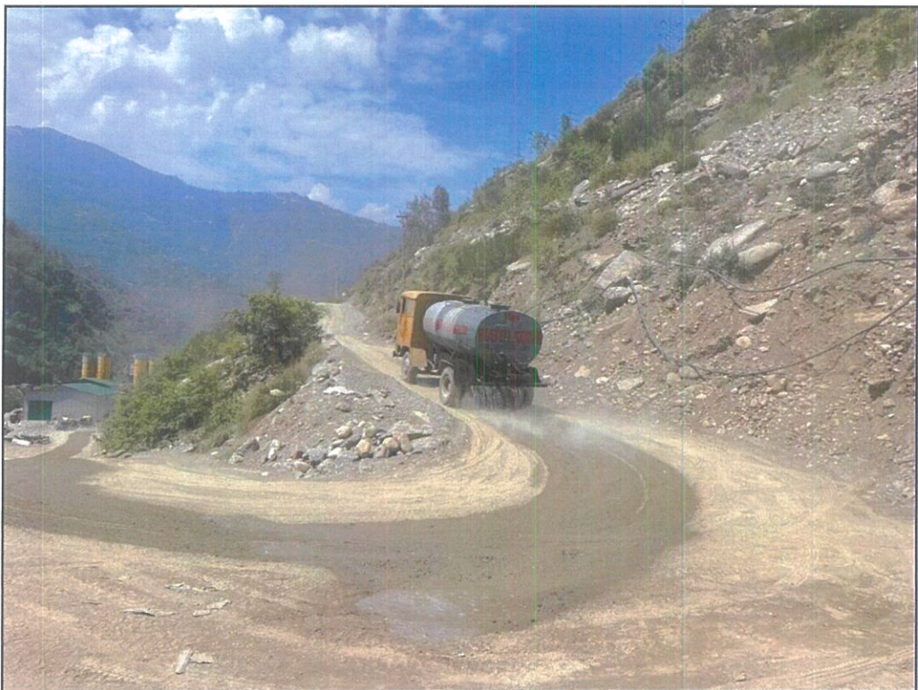
Picture-2. Water Tanker sprinkling water in Moin Road.
