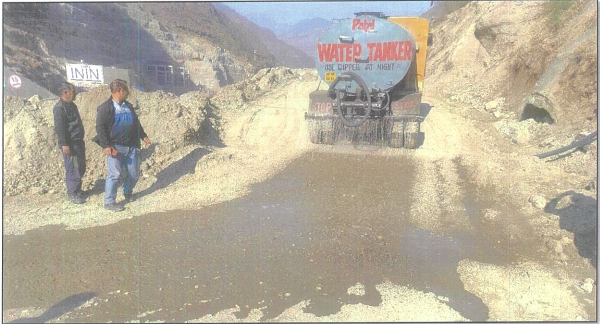
Water sprinkling at work site & NH 05.
