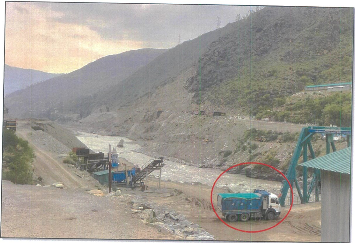
Picture-5. Dumper covered with net to avoid dust emission.
