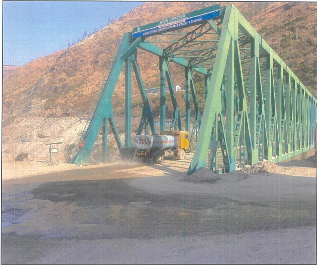
Picture-1. Water Tanker sprinkling water on site.
