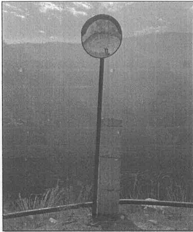
Picture-5. Convex mirrors installed.
