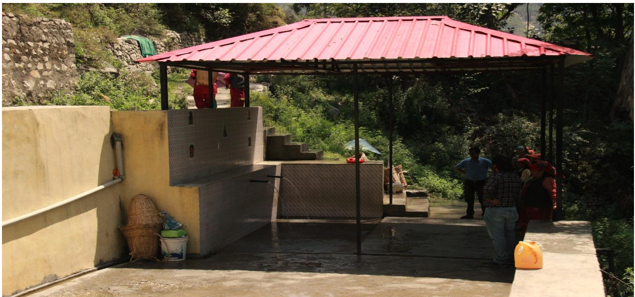
Figure 5-16: Rain water harvesting structure at Rampur
