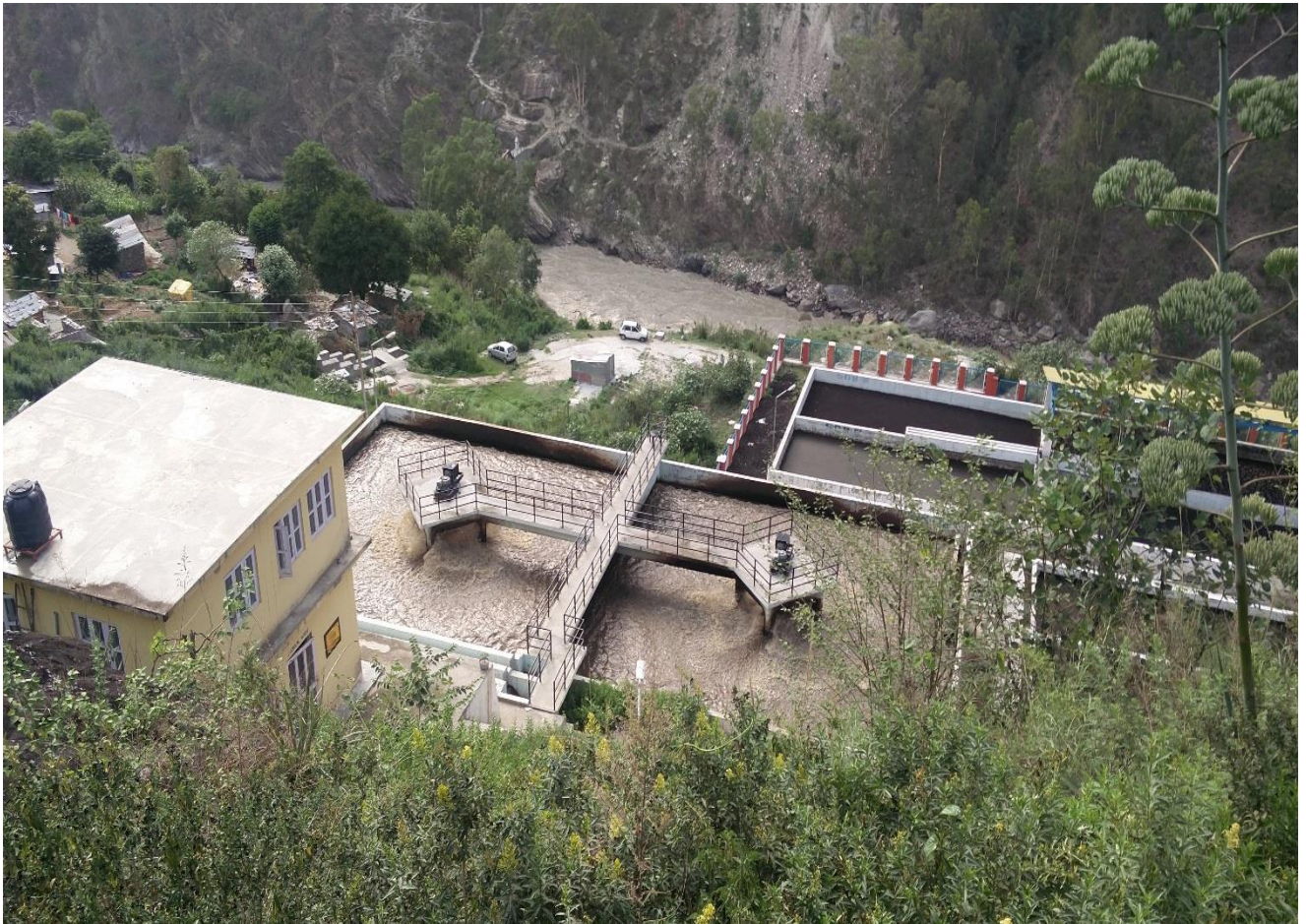
Figure 5-17: STP constructed by SJVN Limited at Jhakri
