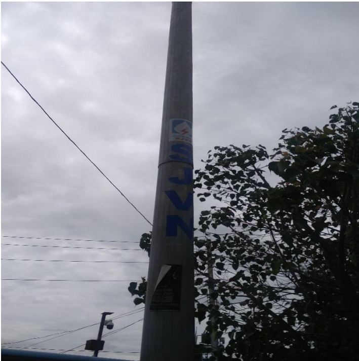
Installation of high mass light in MC Shimla
