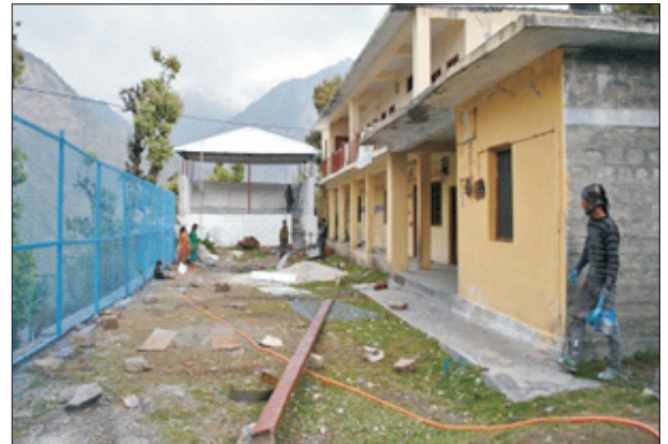
Chain link fencing around the Panchayat Complex Ponda
