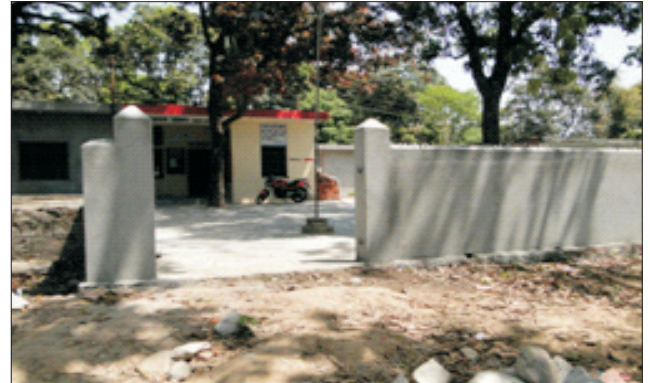
Boundary Wall at Gram Panchayat Jaangal
