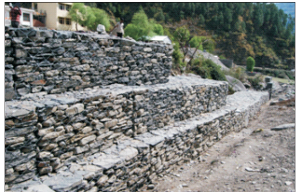
Retaining wall at GSSS, Showad
