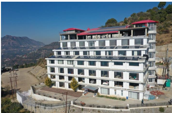
Figure 36: IAMD Building at Solan
