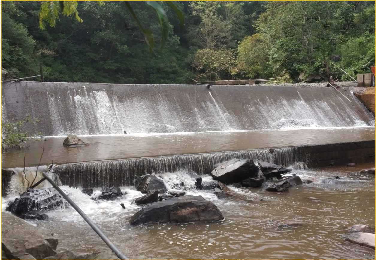
Figure 27: Checkdam constructed at Gount Khad
