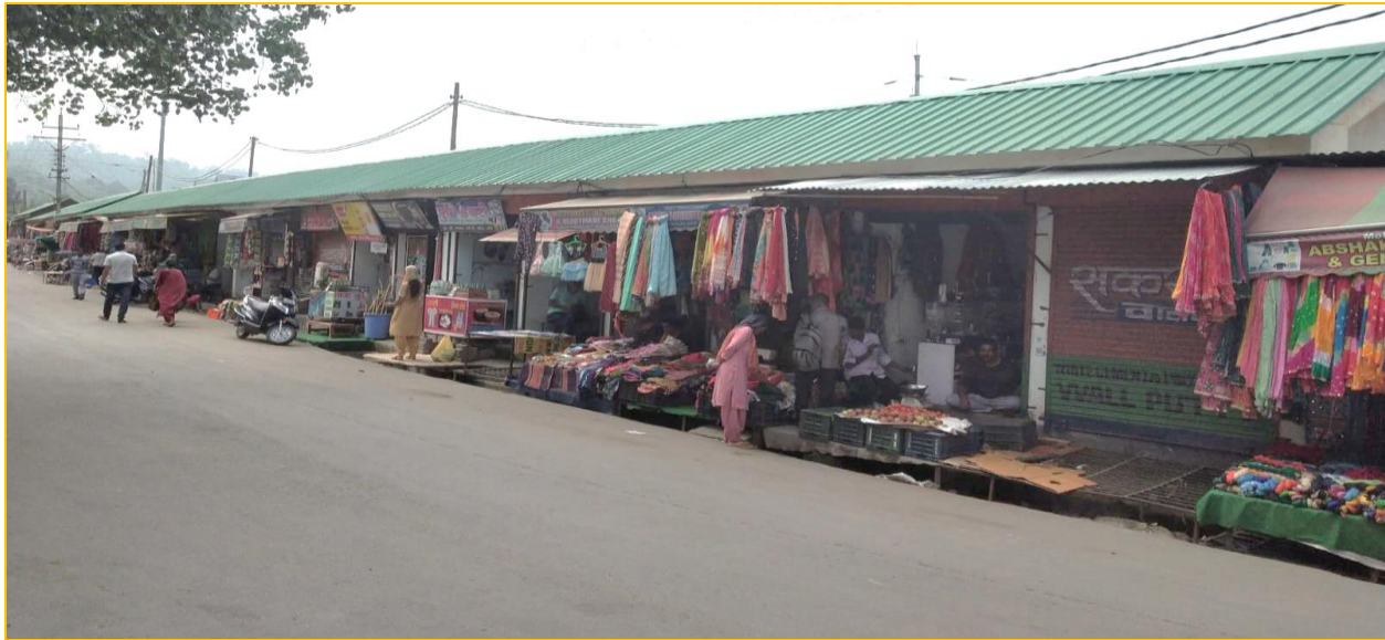
Figure 39: Shops constructed at Sujanpur bus stand
