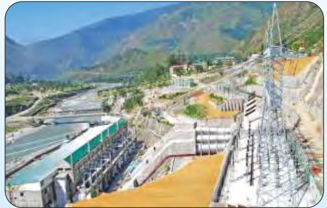
412 MW - RHPS (Power House)
