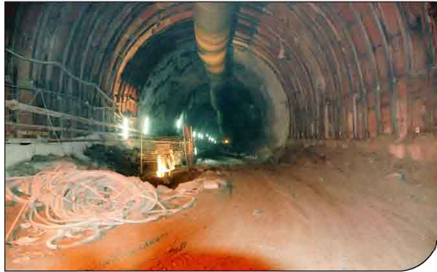
Tunneling work of Rampur Project in progress
