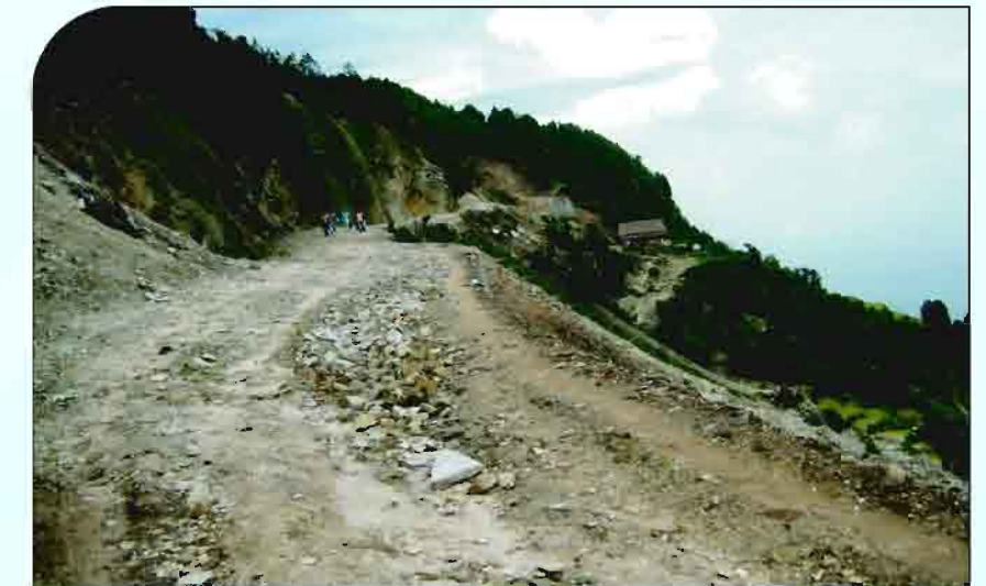
Takeoff point of access road for PH & TRT - Arun-III Project
