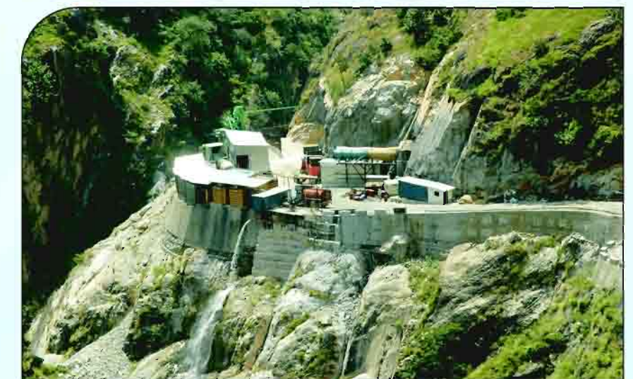
An adit of Rampur Project
