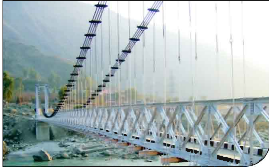
Construction of Bridges in project area
