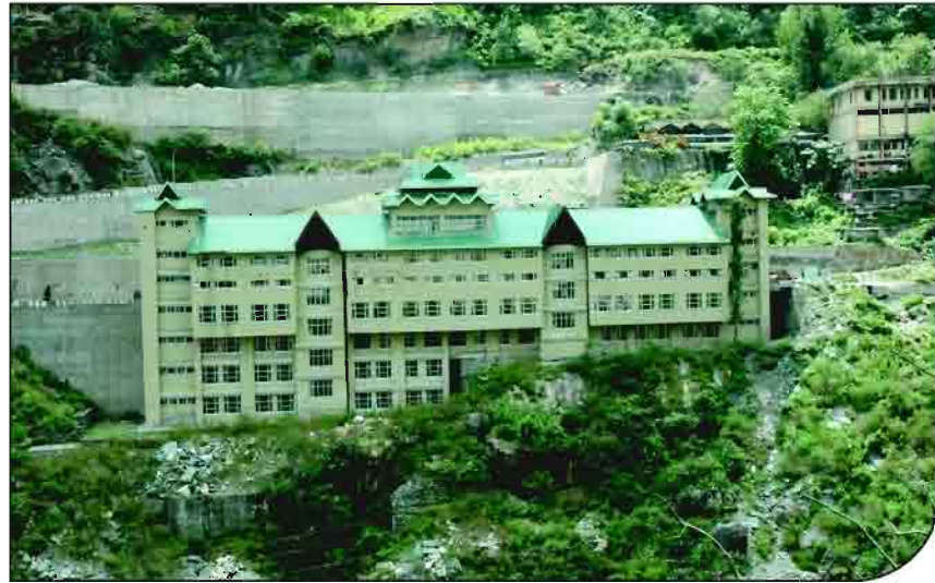
SJVN assisted bus stand under construction at Rampur
