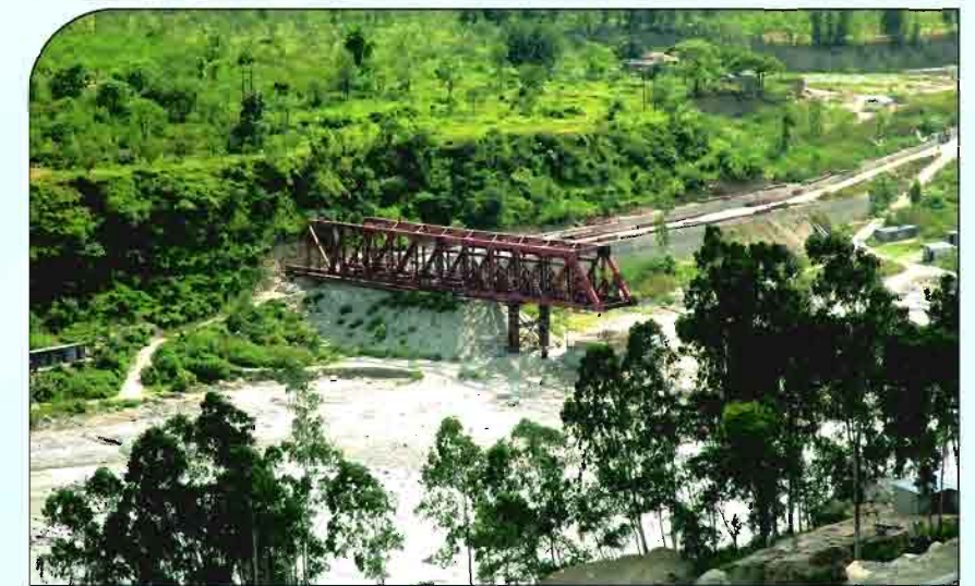
Construction of Bridges in project area
